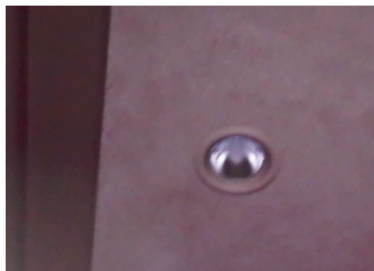
After air sealing lights, blow cellulose insulation without voids, gaps or compression over all IC rated light fixtures.
